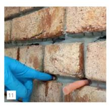
After cutting, the rods are pushed back 2-3 cm into the wall. The rods remain inside the wall.
