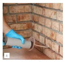
Clean the holes with KÖSTER Drill Hole Cleaner or flush with water.
