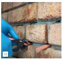
After applying the injection, the capillary rods remain in the masonry. Protruding ends are pulled out and cut off.
