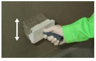
After the material has cured, the KÖSTER Restoration Plaster Key is splashed onto the substrate so that the plaster key is no thicker than 5 mm and covers approximately 50 % of the area. This step will ensure the optimal adhesion of the KÖSTER Restoration Plaster.
