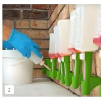
Remove cartridges after this period, empty cartridges can be removed immediately.
