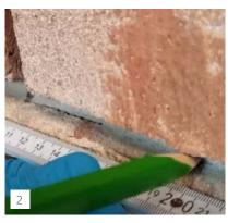
In case of a 50 cm wall thickness the drill hole spacing is 10 cm (see Technical Data Sheet).
