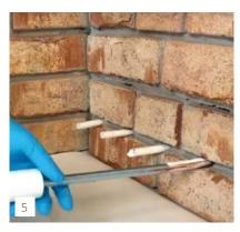
The length of the capillary rods must be at least 7 cm longer than the depth of the drill hole. Measure and cut the capillary rods accordingly.
