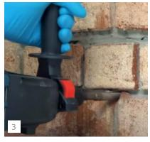
Drill horizontal holes (14 mm diameter) according to the table overleaf in the lowest horizontal joint with a depth of 5 cm less than the thickness of the masonry.
