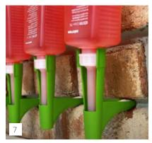
Place the KÖSTER Crisin 76 cartridge in the suction angle's clamping device, so that the supply tank fills up with KÖSTER Crisin 76.
