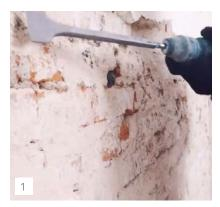
First the old damaged plaster is removed from the masonry
