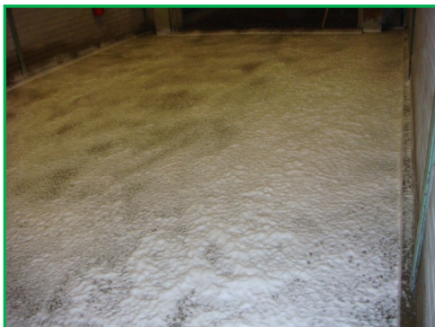
Pic. 12: KÖSTER ORC D detergent applied with the foam gun
