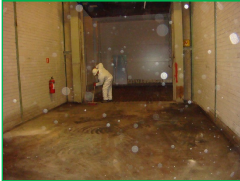
Pic. 8: Removing the coarse dirt with a broom
