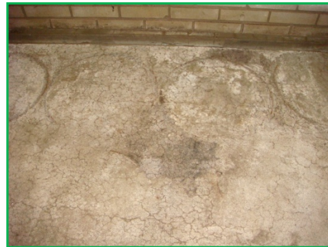
Pic. 16: Clean surface & open capillaries after 3x spinning of KÖSTER ORC D and vacuuming of the left water.
