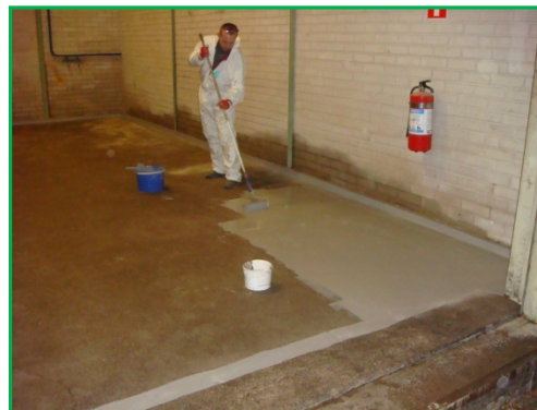
Pic. 18: ...blocking any further migration of the oil to the surface.
