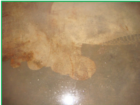
Pic. 10: Turbo Jet washed floor (top) & unwashed floor (bottom)
