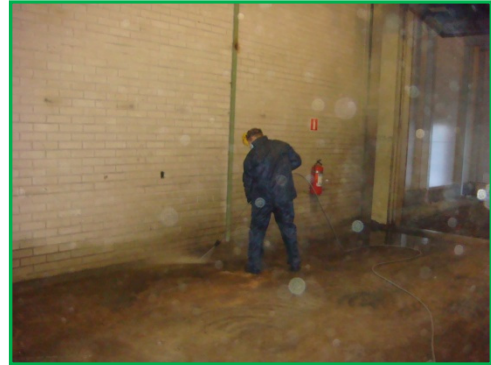
Pic. 9: Turbo Jet washing with hot & high pressured water (100°C, 300bar)
